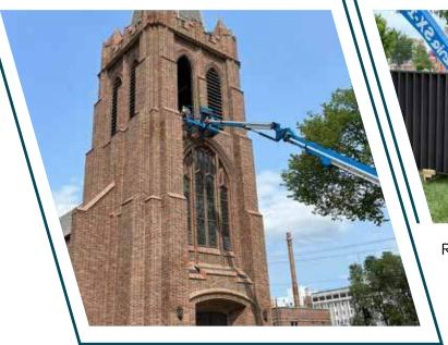
Replacement of 8 well-worn louvers with 8 new ones in the Bell Tower. Our thanks to Industrial Builders for their work in the removal and replacement of the louvers, and to Tim Ellenson for sharing his gifts and talents by caulking each of the louvers.
